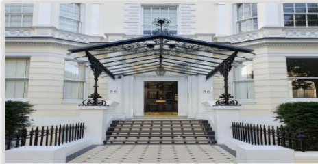
INTERNAL COMMUNAL REFURBISHMENT
